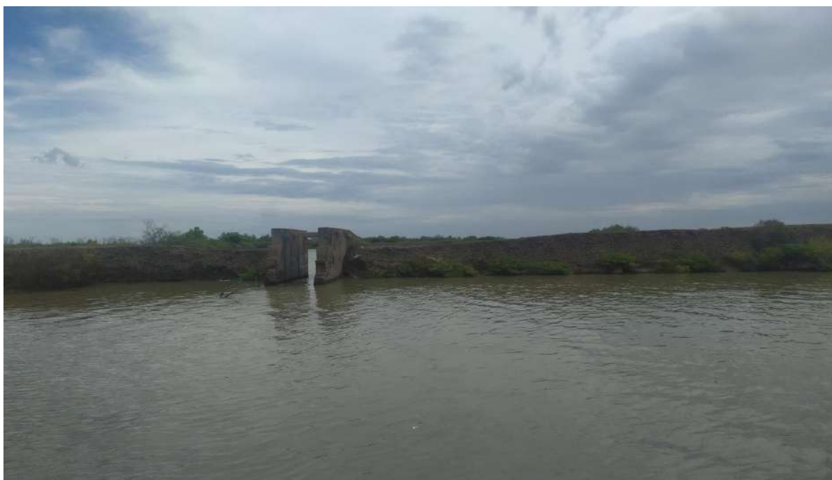
Photo 6.5: Aquaculture effluents are connected in the Mangroves in Thillaivilagam
