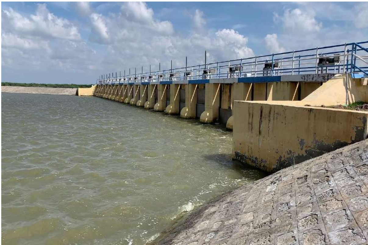
Photo 6.1: Shutter Construction in Valavanar River at Munnangadu
