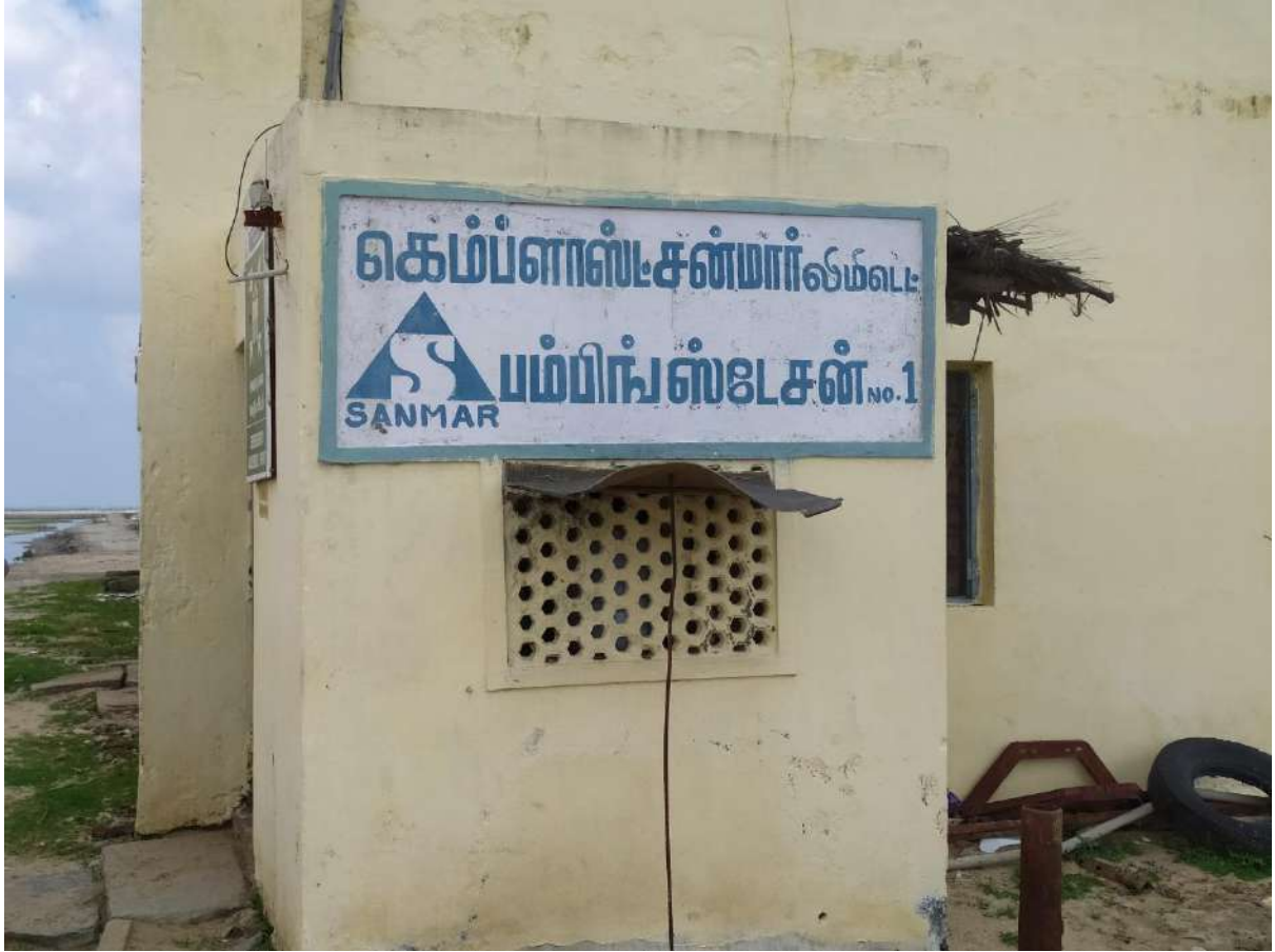
Photo 6.2: Chemplast pumping station in Kodiayakadu
