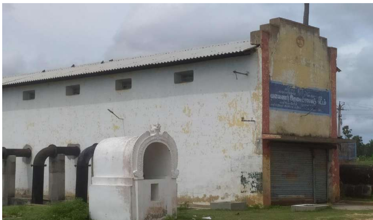
Photo 3.1: Irrigation Pumping Station in Annapettai
